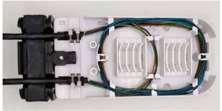
Drop Cable Installation
